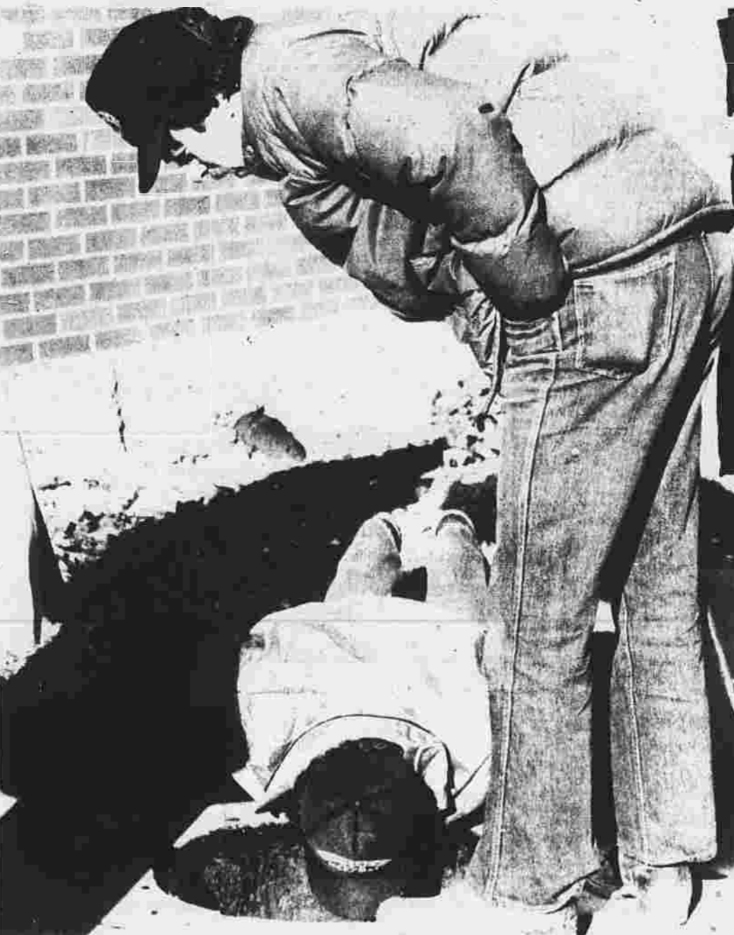
Ed Alexander of the Hazardous Waste Disposal Unit of the state Department of Environmental Protection looks into a manhole near the Multi-Circuits manufacturing plant this morning while Brian Coss of the DEP looks on. DEP workers
